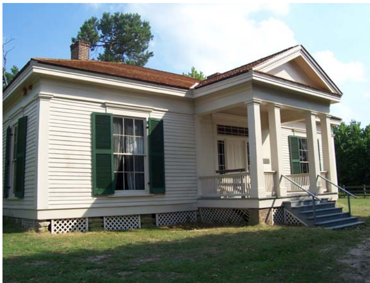
We'll be excavating in the backyard of the Royston House at Historic Washington State Park this November in order to help reconstruct the back porch and to identify 19 th century outbuildings.
